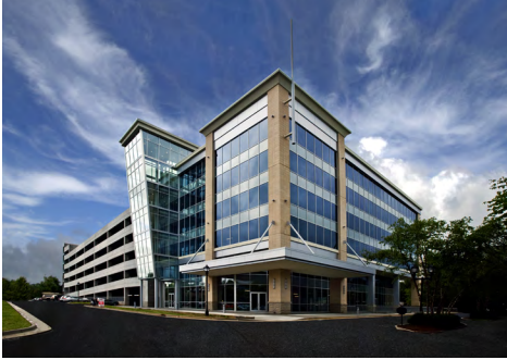
Perimeter Town Center
